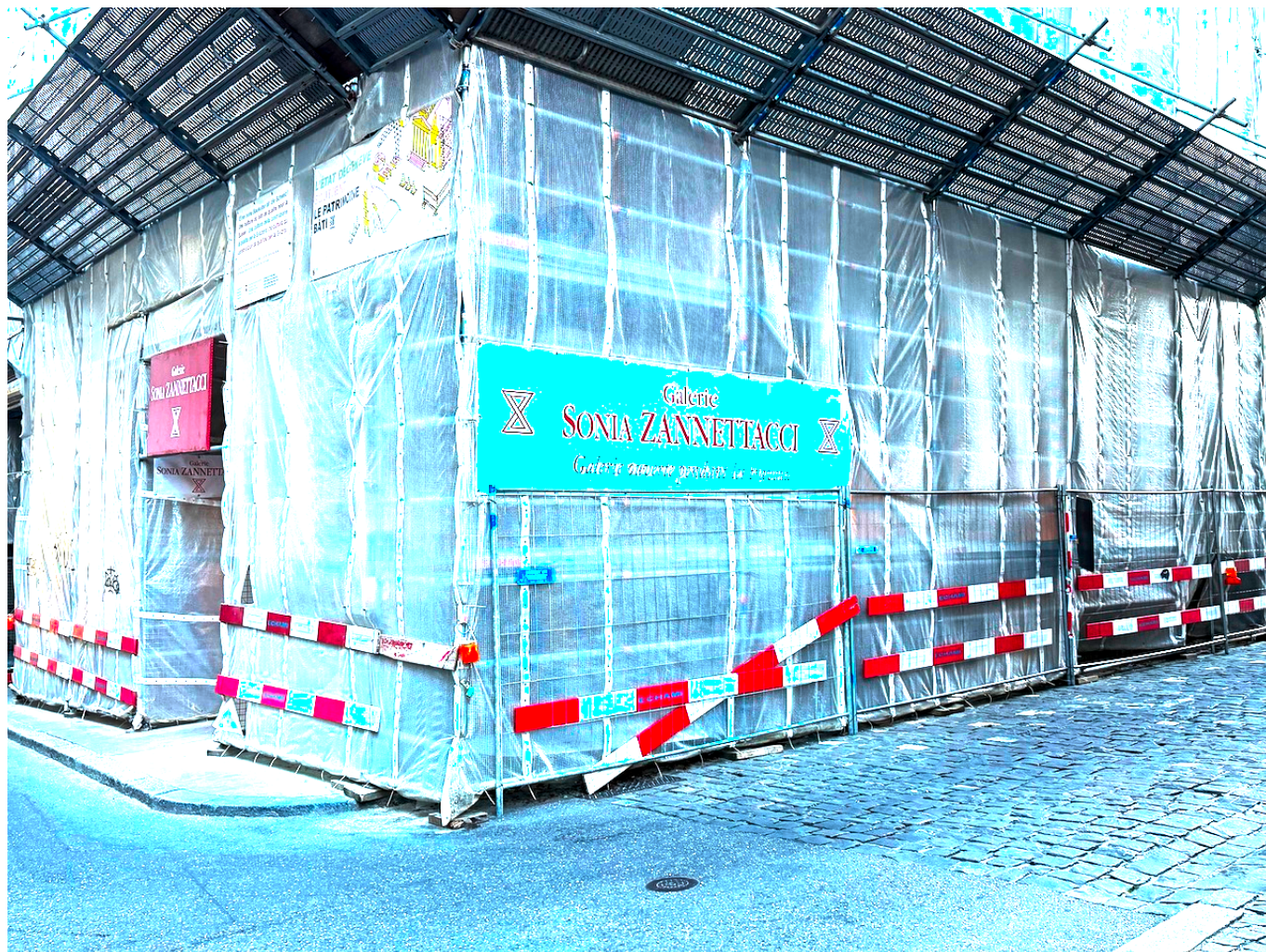
The façade of the new gallery is still behind scaffolding... Photo © N. Sikorsky
